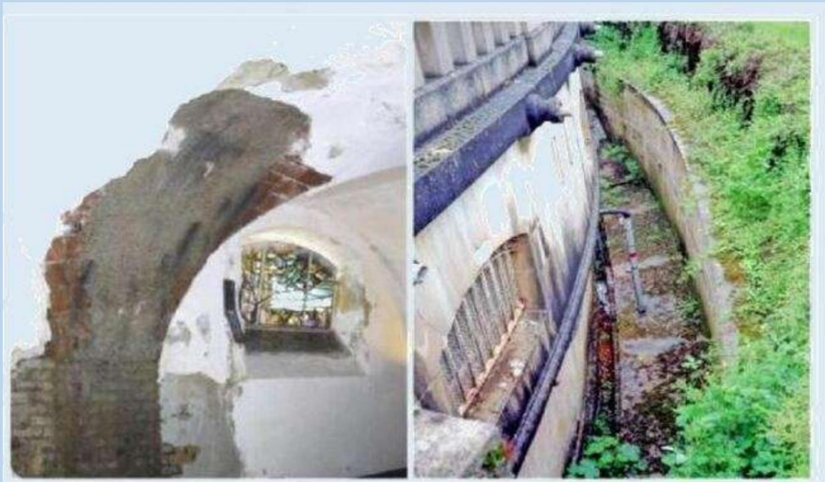
Damage to the crypt due to infiltration
