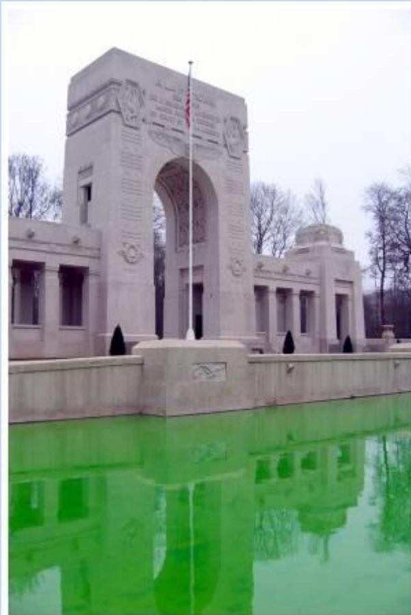
Leak test of pavilions (2006)
