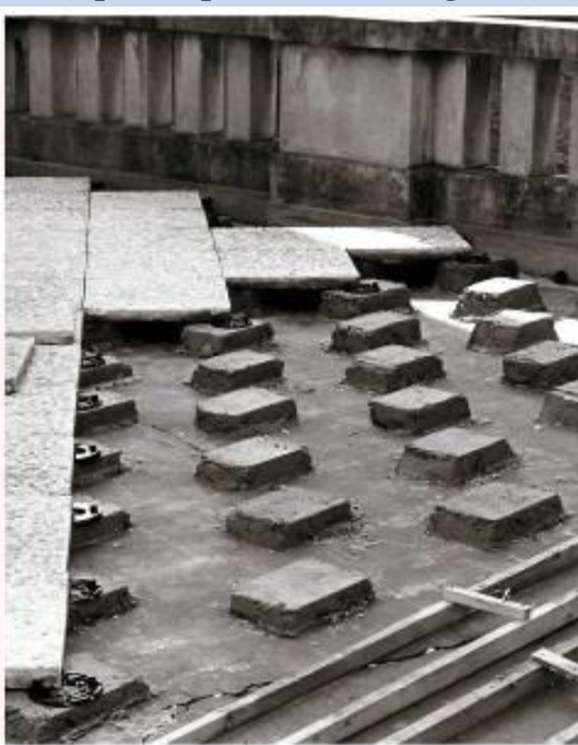
Slab and plastic pedestal cladding (1980)
