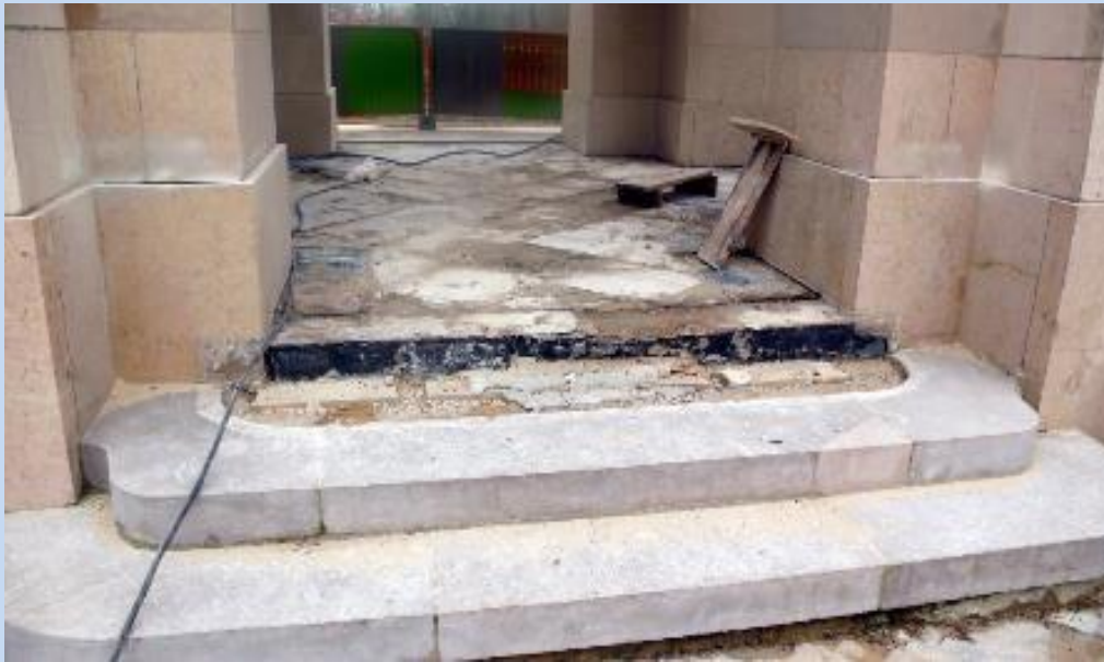
Sealing work under the gantries
